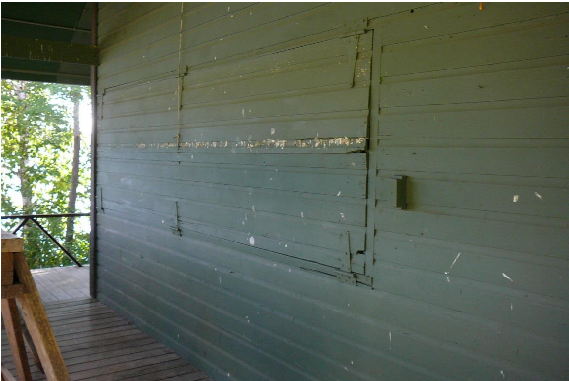
Photo 8. View of typical double top and bottom hinged shutters on east elevation of Beenadeewin (#1).
